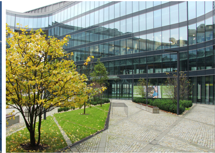
REPUBBLICA CECIA OSTRAVA, NOVÁ KAROLINA PARK OSTRAVA - STRATOBEL STOPRAY 66.2 E STRATOBEL STOPRAY 66.2 - CMC ARCHITECTS - BREEAM VERY GOOD
