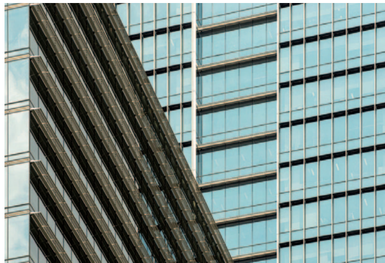
SINGAPUR SINGAPUR, TANJONG PAGAR CENTRE - STOPSOL SUPERSILVER CLEAR A STOPRAY VISION-37T - SKIDMORE, OWINGS & MERRILL (SOM) USA & ARCHITEKT 61 PTE LTD - LEED PLATINUM
