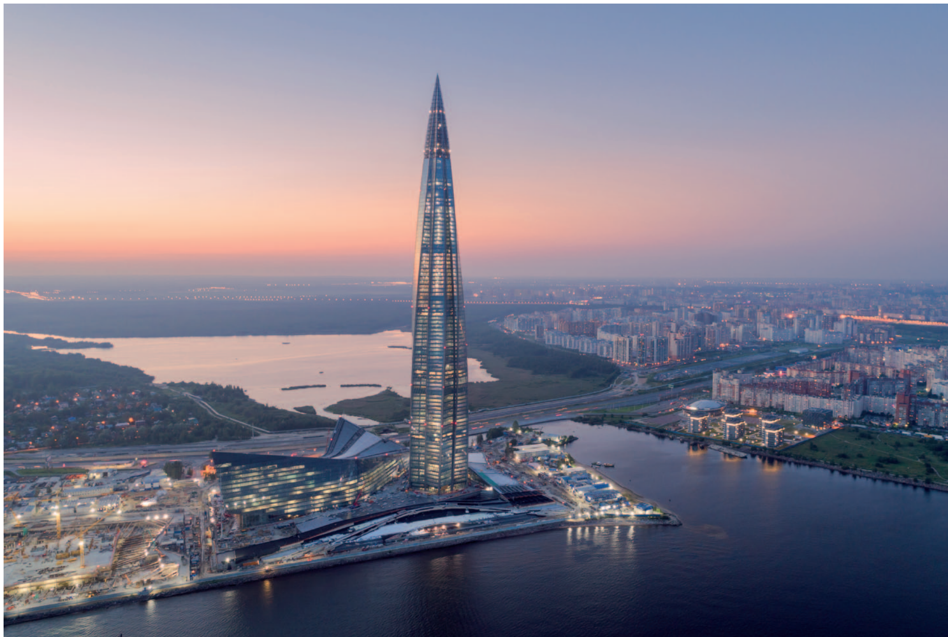
RUSKO SAINT PETERSBURG, LAKHTA CENTRE - ENERGY 72/38, IPASOL BRIGHT WHITE ON CLEARVISION A PLANIBEL LINEA AZZURRA - TONY KETTLE A GORPROJECT CJCS - LEED PLATINUM
