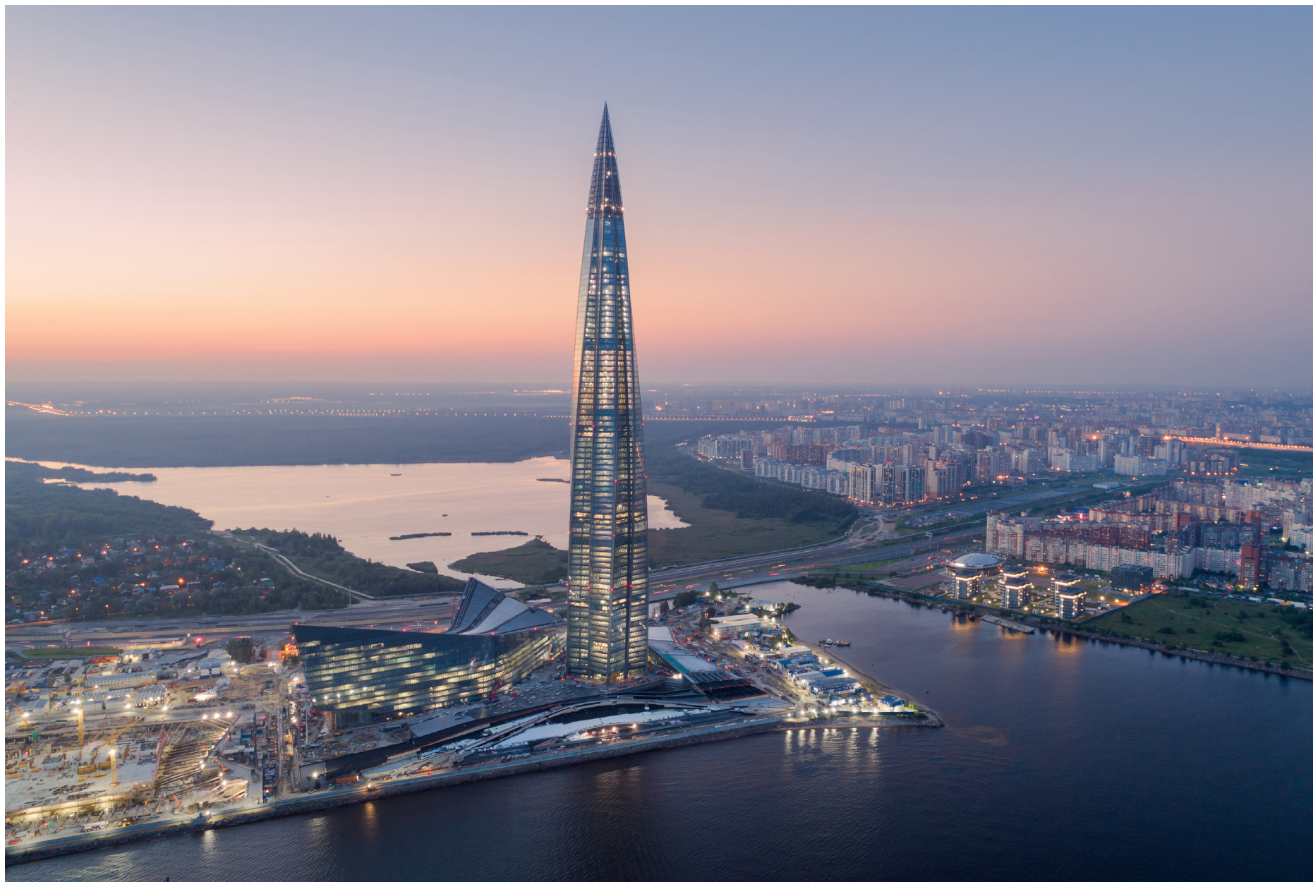
RUSLAND ST. PETERSBURG, LAKHTA CENTRE - ENERGY 72/38, IPASOL BRIGHT WHITE ON CLEARVISION EN PLANIBEL LINEA AZZURRA - TONY KETTLE AND GORPROJECT CJCS - LEED PLATINUM
